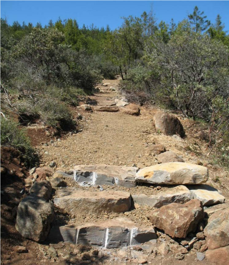
Photo 25.5 - Trail Reconstruction Project: After
