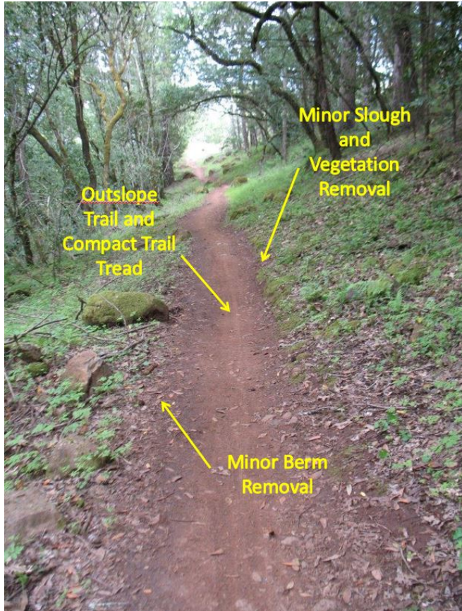
Photo 25.1 - Trail Requiring Light Tread Maintenance
