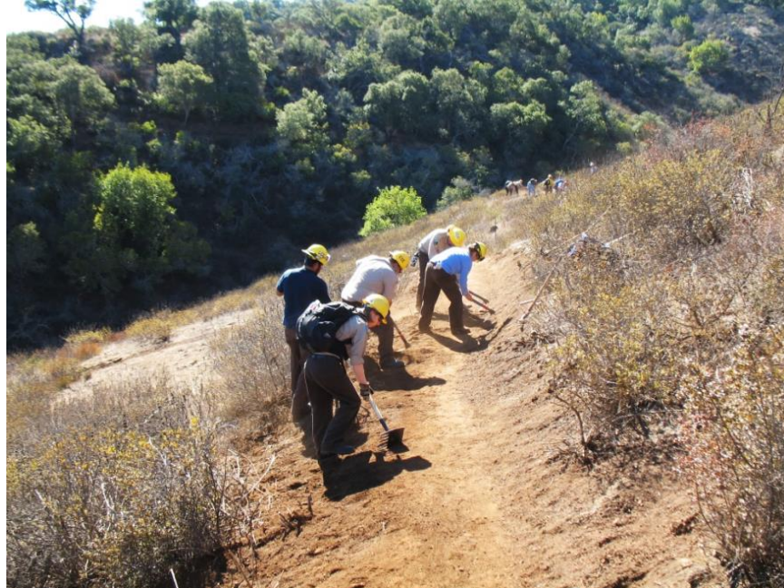
Photo 25.3 - Crew Performing Trio Maintenance After Brushing
