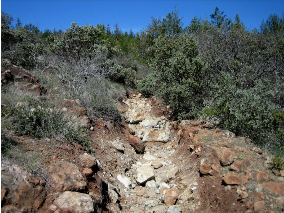
Photo 25.4 - Trail Reconstruction Project: Before
